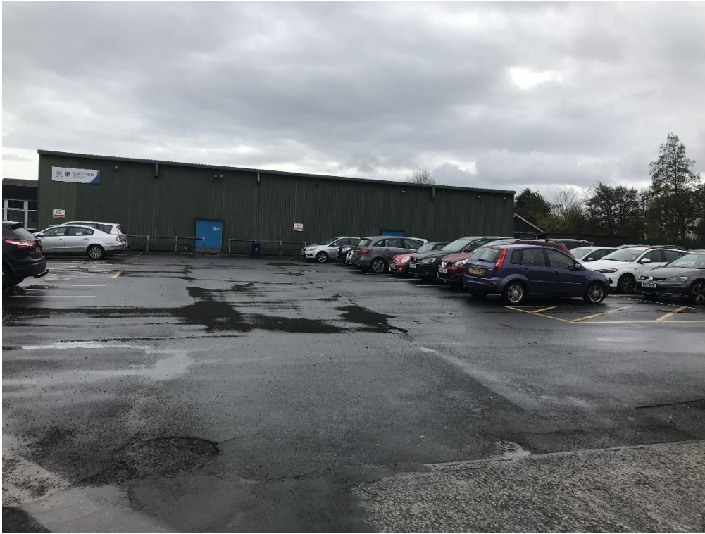
Photo 3: View showing carparking area in the south of the site.
